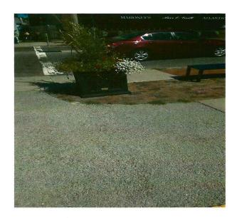
Perk-Crete pavement in downtown Orleans handles pedestrian traffic and intercepts surface water during storm events to provide needed drainage
