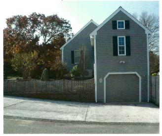
Perk-Crete pervious parking area for residents eliminates ponding and keeps storm water on-site
