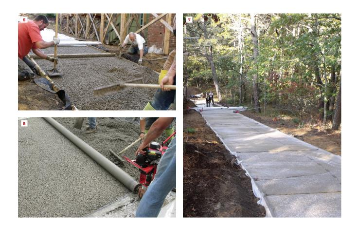
ride on top of the forms. After screeding the concrete flat, radius edging tools softened the edges of the driveway along the forms.
